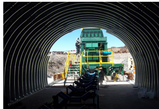
(Left) Crews install a conveyor belt to the Floats Bin. (Below) A view through the tunnels which will be placed underground.
