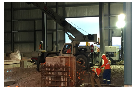
Work continues for the Mill Building. Equipment installation begins in December.
