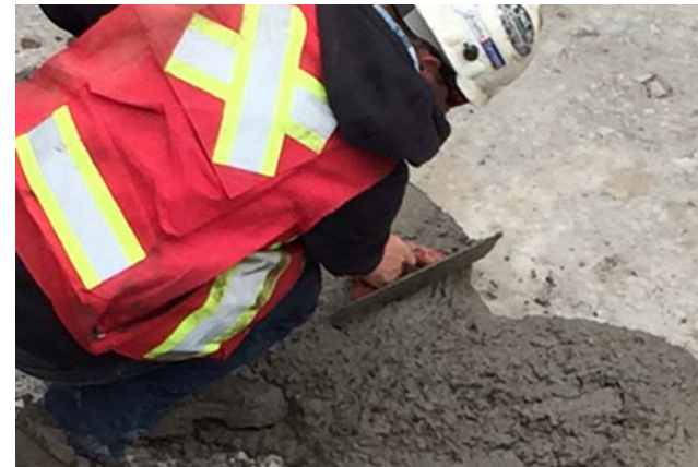
Concrete is being smoothed and shaped for the mud pack. A five-dollar bill, placed by CFI CEO Lindsay Gorrill, was covered for good luck, a tradition for the first concrete pour of mining and construction companies.
