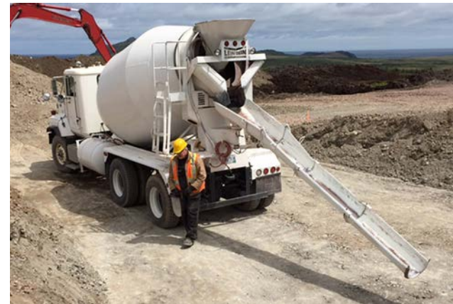
Workers prepare to pour first concrete at CFI facilities. The concrete – or ‘mud pack’ – is a base for the new mill raft, which is the base for the building where the new ball mill will be placed.
