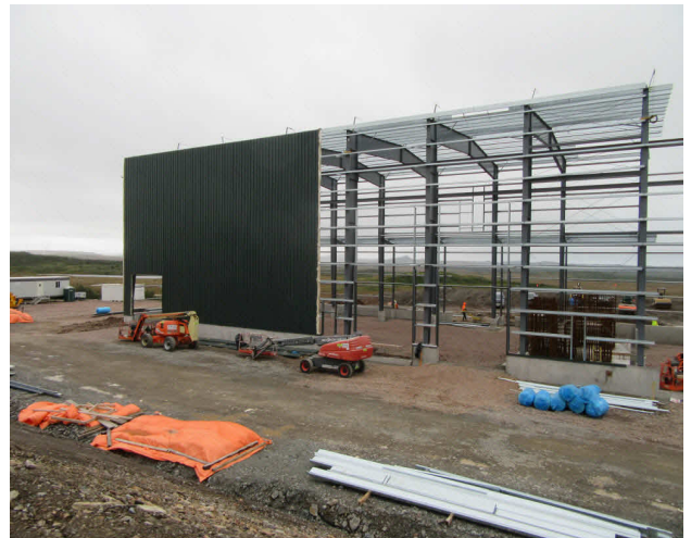
Mill building is in the process of being sheeted as the final steel erection progresses.
