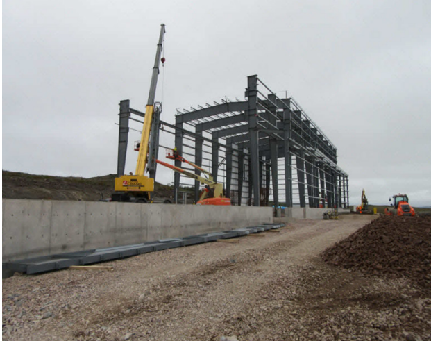
Work continued on the mill building steel throughout the month
